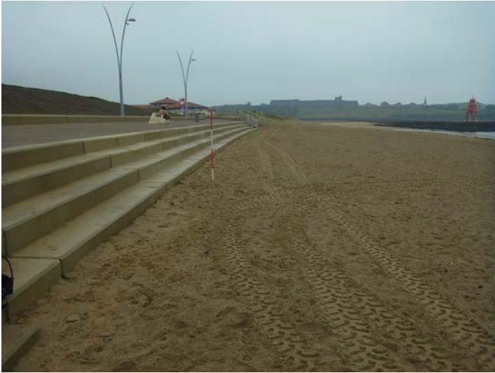
Plate 1 – Survey photograph 1bSS2_20140428_N2.JPG
