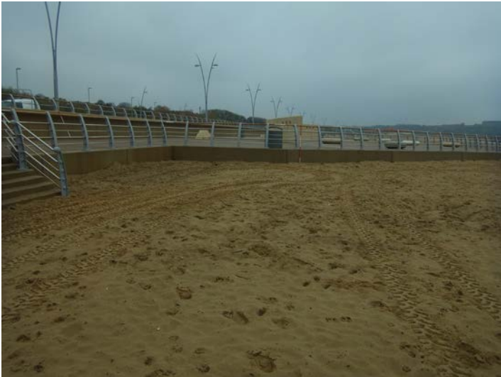
Plate 3 – Survey photograph 1bSS4_20140428_N2.JPG
