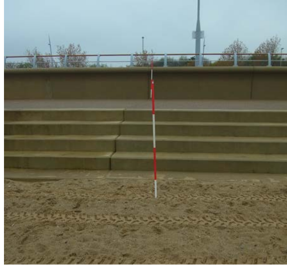
Plate 2 – Survey photograph 1bSS3_20140428_Up1_N2.JPG
